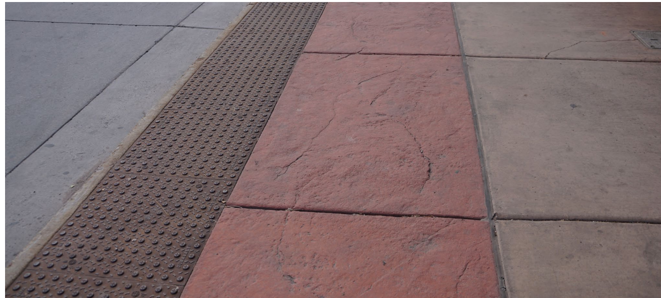
Figure 32: Ground Mounted Tactile Strip
