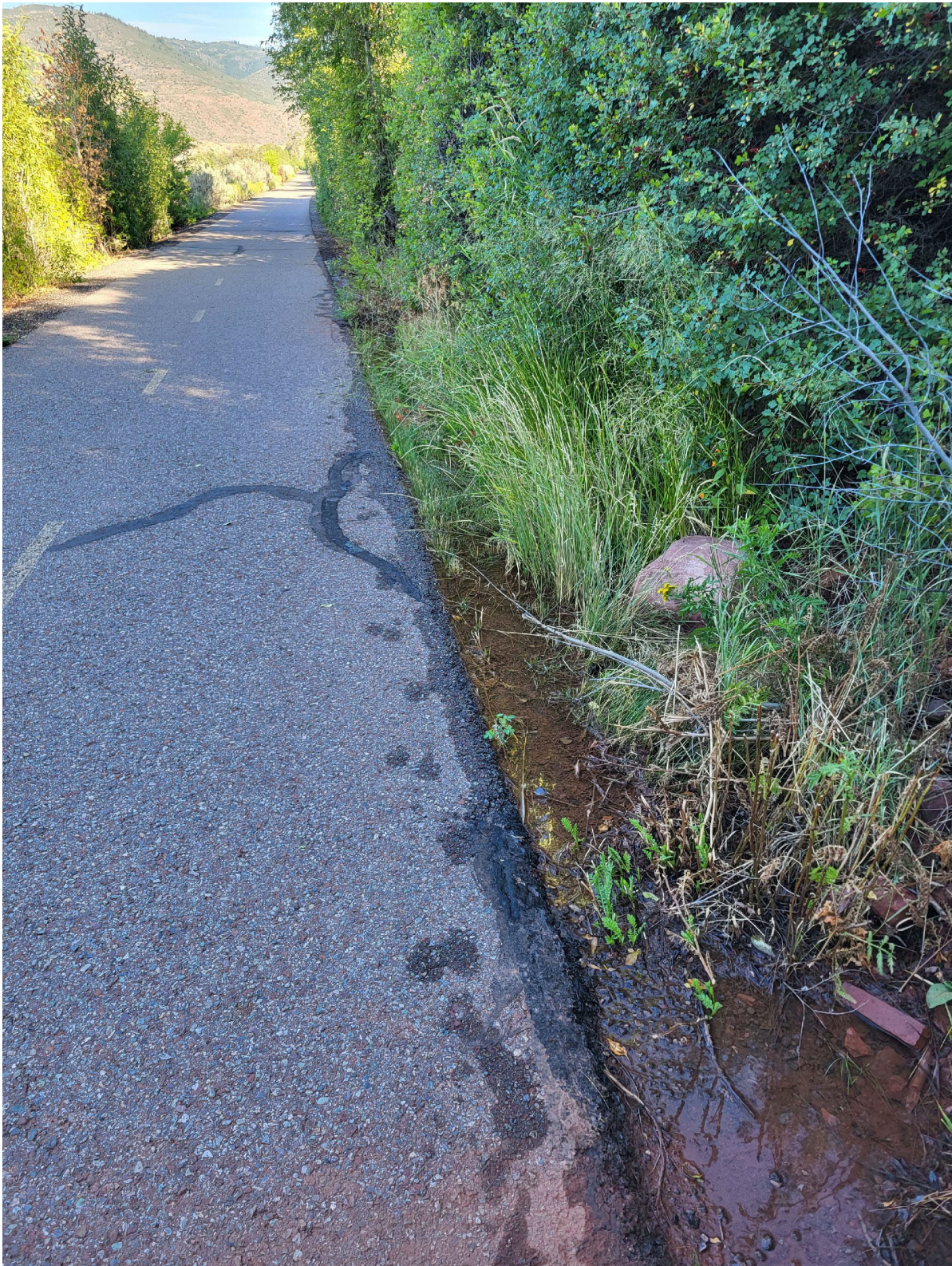
Photo – water along RGT shoulder, leaking from Thompson Glen Ditch
