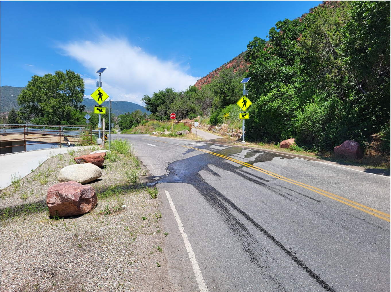
Photo – water from Thompson Glen Ditch running over CR 154. The water is leaking out of the ditch, goes under the RGT and then down to CR 154
