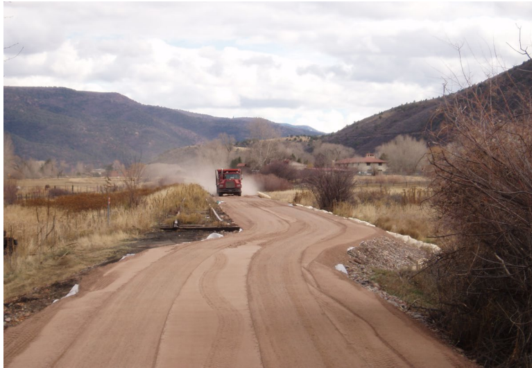
Carbondale to Catherine Store Trail Segment Under Construction
