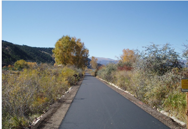
Newly Constructed Asphalt Surface Trail Segment near Emma
