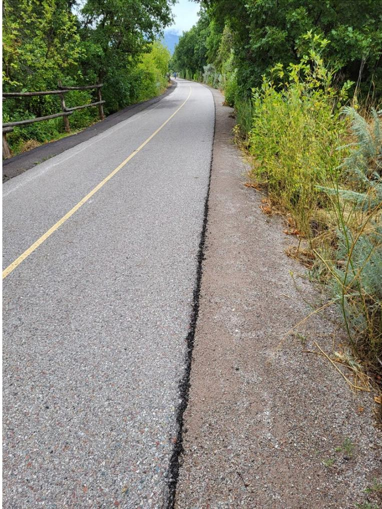
**Photo 3 – newly placed and compacted shoulder on left side of photo; old shoulder in need of more gravel on right side (project aims to fix)**
