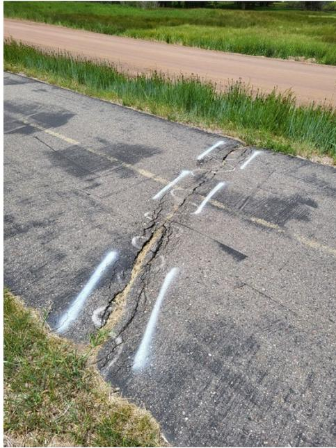
**Photo 1 – full width crack**
