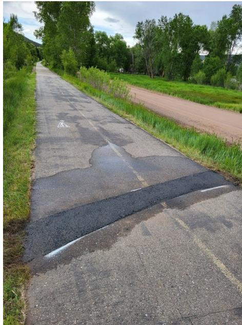
**Photo 2 – crack from “Photo 1” has been repaired! (along with several others)**
